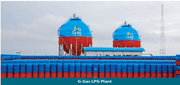
G-Gas LPG Plant
